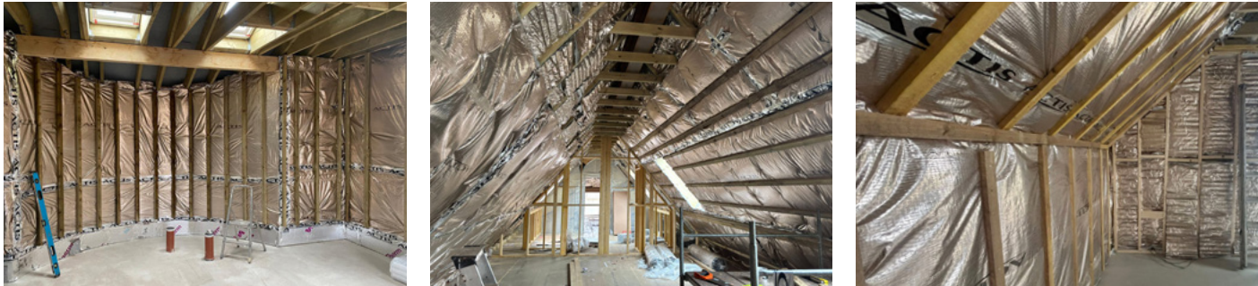
HControl Hybrid as a substitute for Vapour Control Layer in timber pitched roof.
